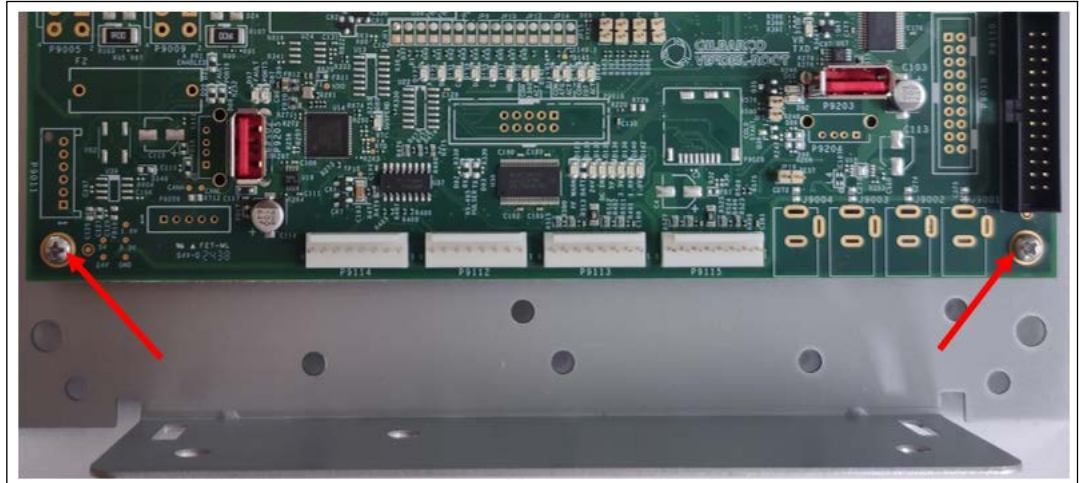
Figure 5-3: Securing the Earth Ground Connection to the PCN
