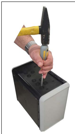
Figure 5-7: Knocking Out Using Hammer
