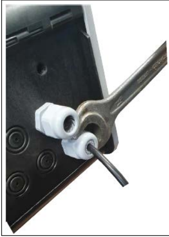
Figure 5-11: Cable Gland Fastening
