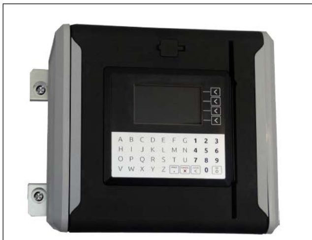
Figure 5-15: Truck PRIME Installed on Truck Wall
