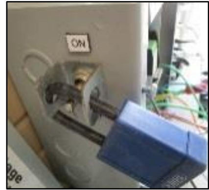
Figure 16: Typical lock-out
