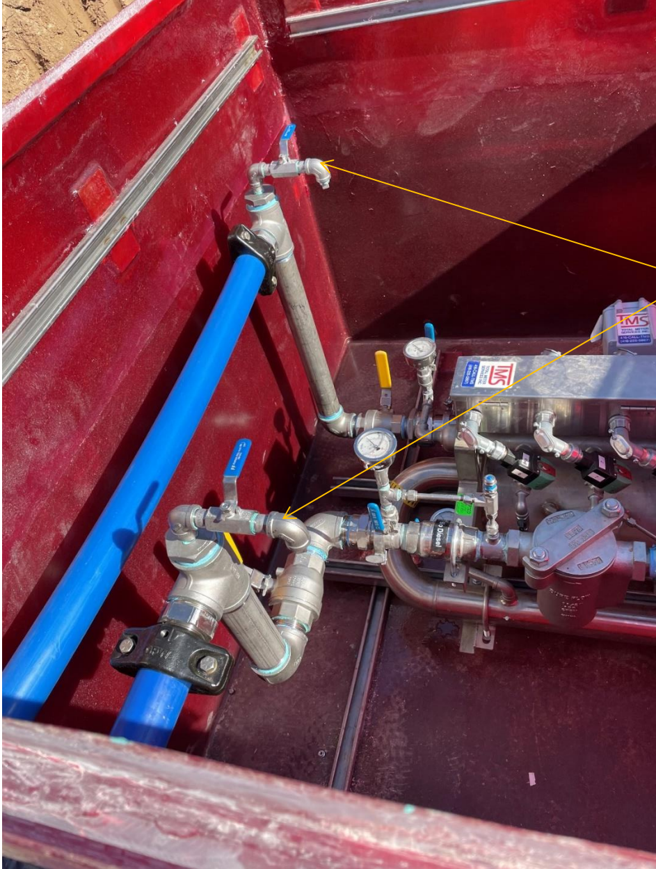
Figure 20: Recommended installation with high point vents
