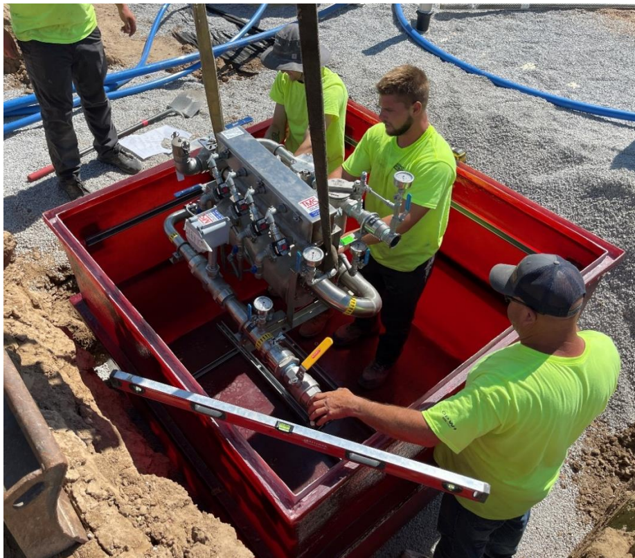
Figure 10: Lowering BBS unit into an underground sump
